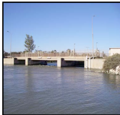
Figure 14 : barrage anti-sel de Fos-sur-Mer (MRM)
