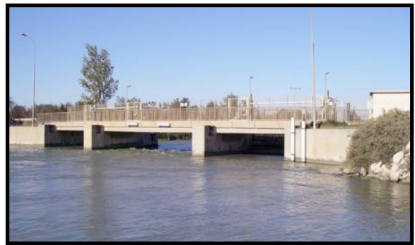
Figure 14 : Barrage anti-sel de Fos-sur-Mer (MRM)
