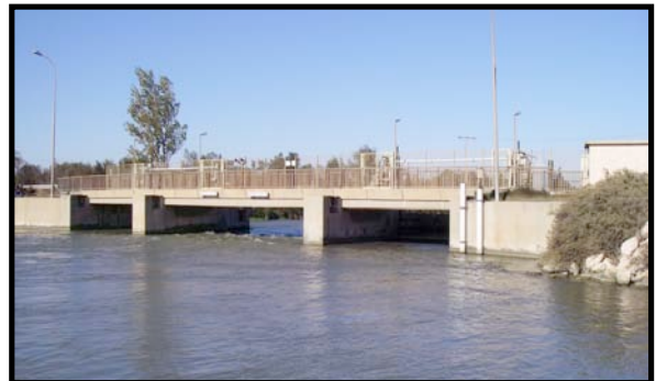
Figure 15 : Barrage anti-sel de Fos-sur-Mer (MRM)
